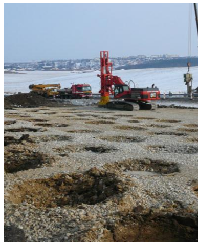
Obr.10: Hutnená pláň Fig 10: Compacted area
