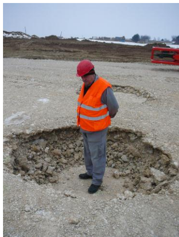
Obr. 9: Depresia po 70 úderoch Fig. 9: Depression after 70 blows
